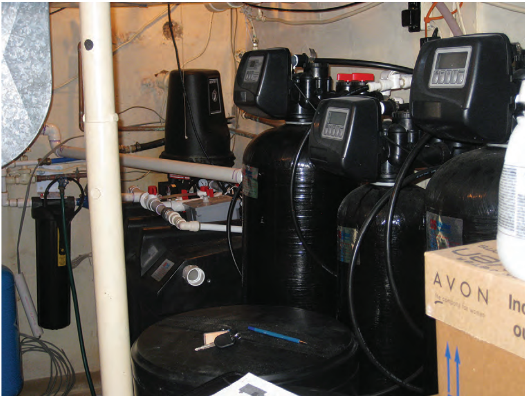
Some arsenic treatment systems can be relatively complex. Pre-oxidation is needed to convert \text{As}^{3+} to \text{As}^{5+} prior to removal by anion exchange. Photograph by Mike Ekberg, Miami Conservancy District.
