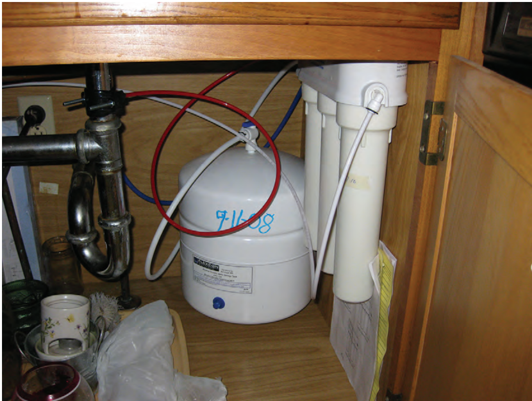
Reverse osmosis is typically part of a single-tap system used to treat just the water used for drinking and cooking. Photograph by Mike Ekberg, Miami Conservancy District.
