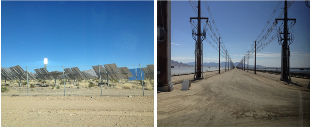
Figure 12. Example linear features, fence and collector lines.
