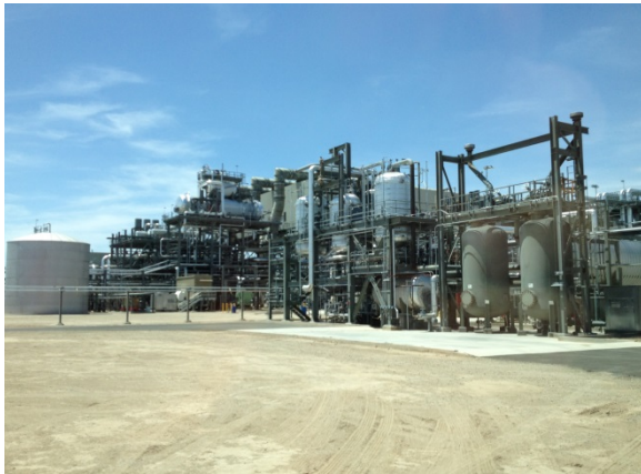
Figure 4. Power generation building.
