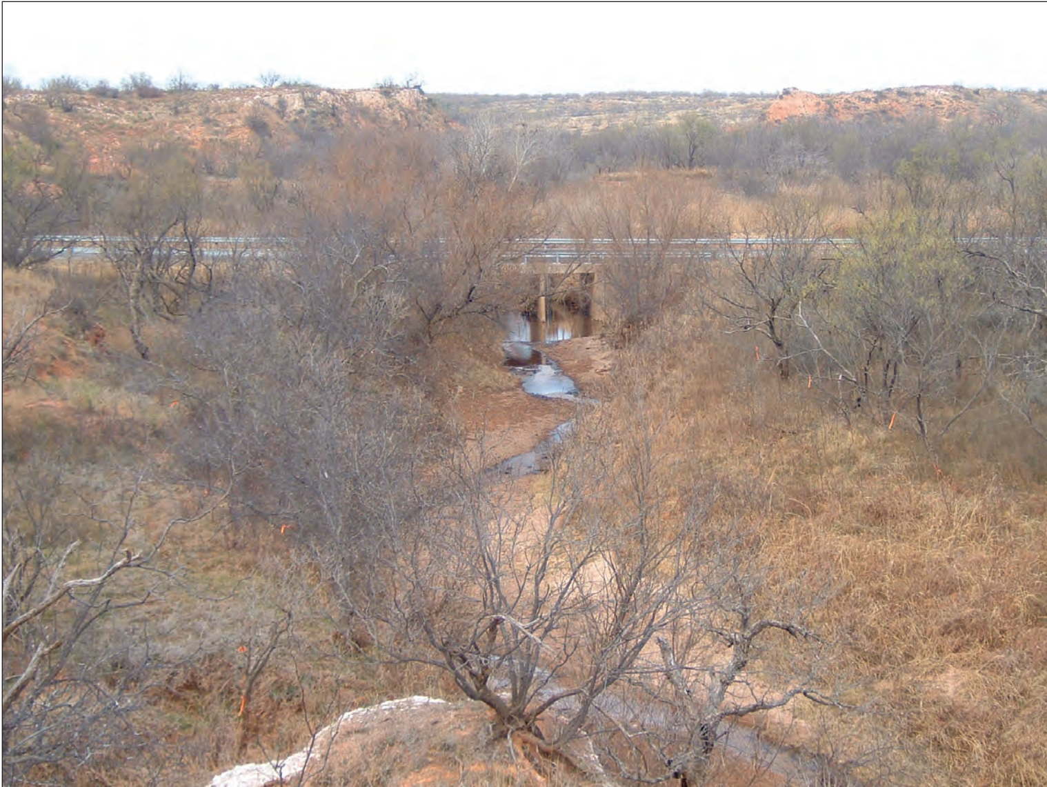
Figure 7. Location of a survey for a slope-area indirect measurement for U.S. Geological Survey station 08080918 in November 2006.
