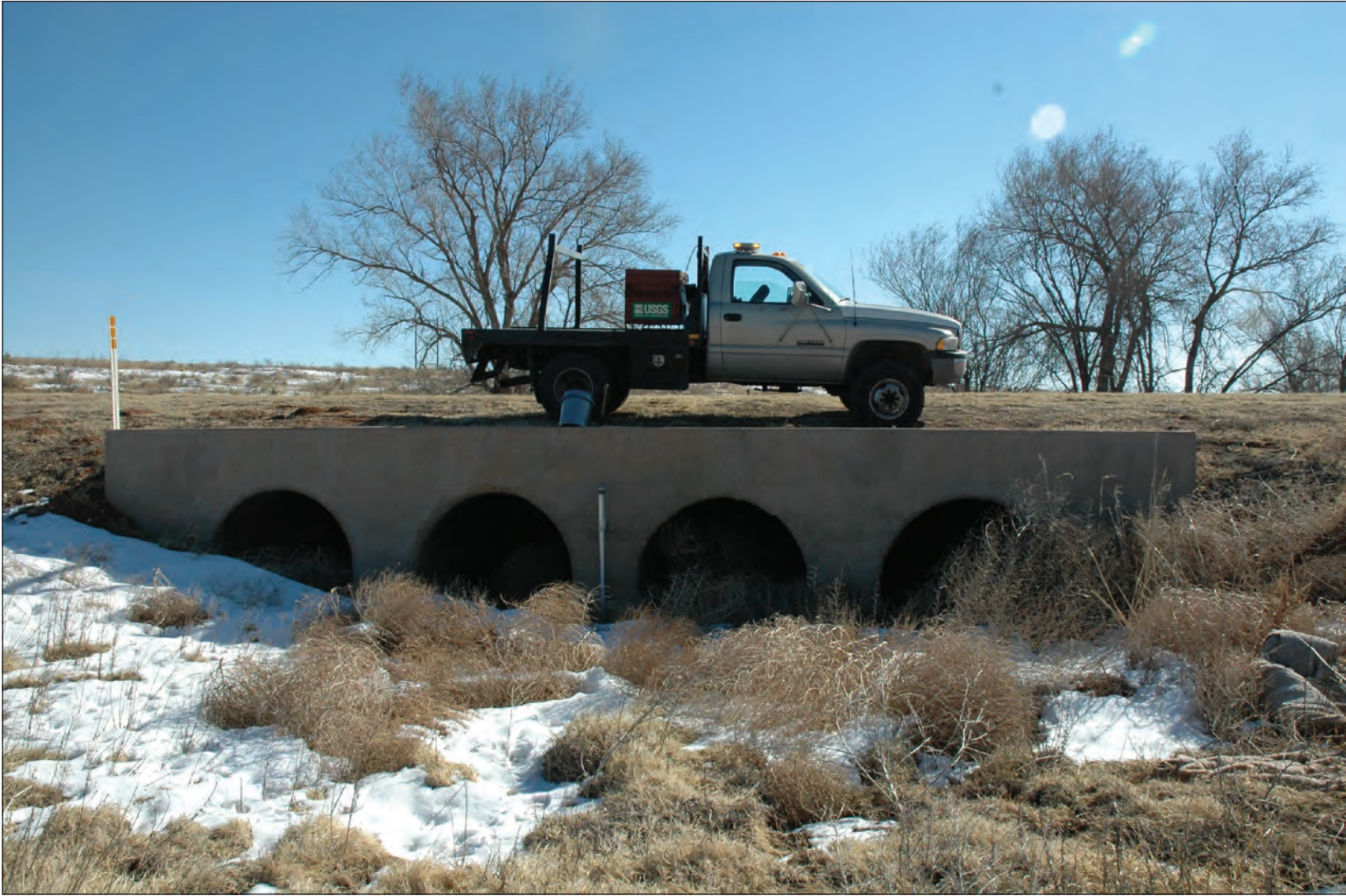
Figure 6. Culvert inlet for U.S. Geological Survey station 08079400 on February 27, 2013.
