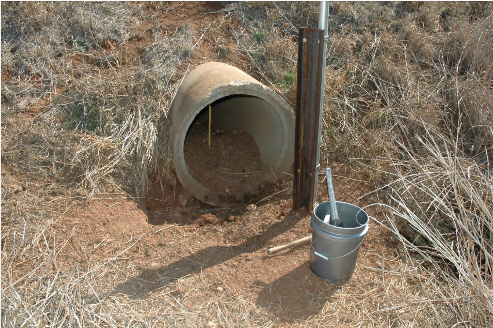
Figure 5. Culvert inlet and crest-stage gage at U.S. Geological Survey station 07299575 in February 2012 during a routine station visit.
