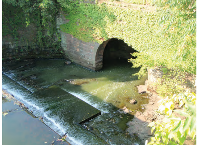
Figure 5. Green algae in Mill River water spilling from Watershops Pond impoundment under the mill at Watershops Pond, Springfield, Massachusetts, September 1, 2010. Photograph by Andrew J. Massey, U.S. Geological Survey.
